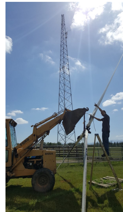
Ken and Casey reattached gear box to casting tower and attached the blades.
