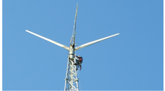
March 16 — Gilbert from Powder River dashes up the wind turbine and ties down the blade to prevent them from spinning.
