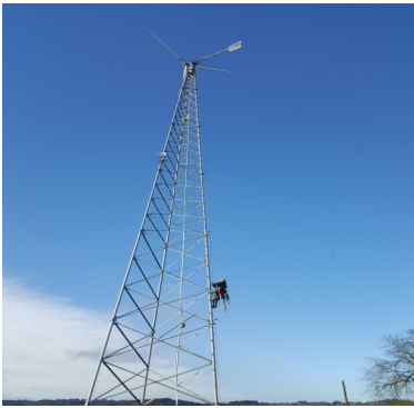
March 16 — Gilbert from Powder River dashes up the wind turbine and ties down the blade to prevent them from spinning.
