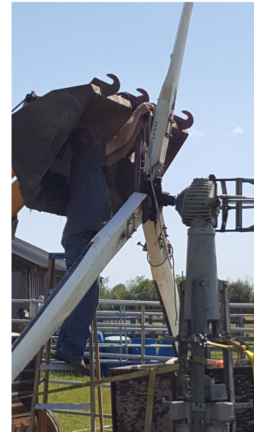
Ken and Casey reattached gear box to casting tower and attached the blades.
