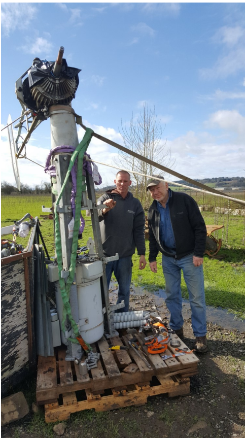
Ken and Casey reattached gear box to casting tower and attached the blades.
