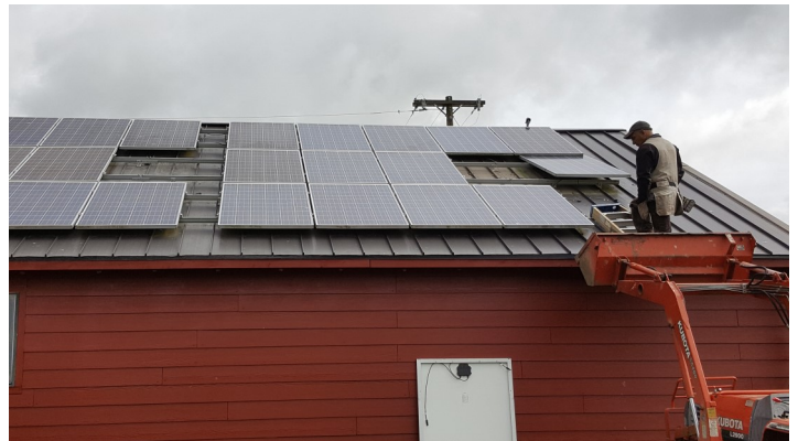
Solar Ki repairing solar panels on shop.
