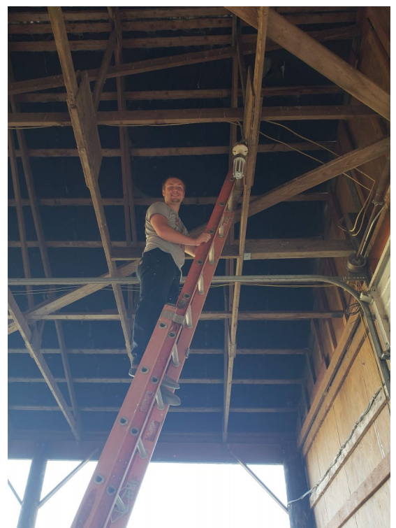
300 watt bulbs (on left) were removed from the sheep barn. They were replaced with 45 watt LED retrofit bulb. Our high school farm assistant, Jared, installed the LED bulbs.
