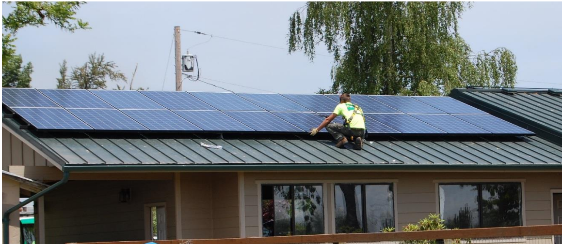
Complete installation of solar panels, May 15, 2013.
