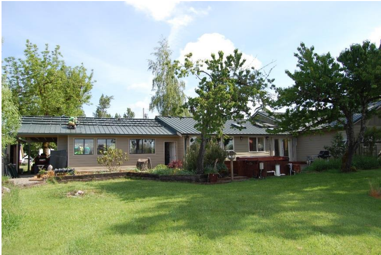
Installation of grid-tied system, May 14, 2013.
