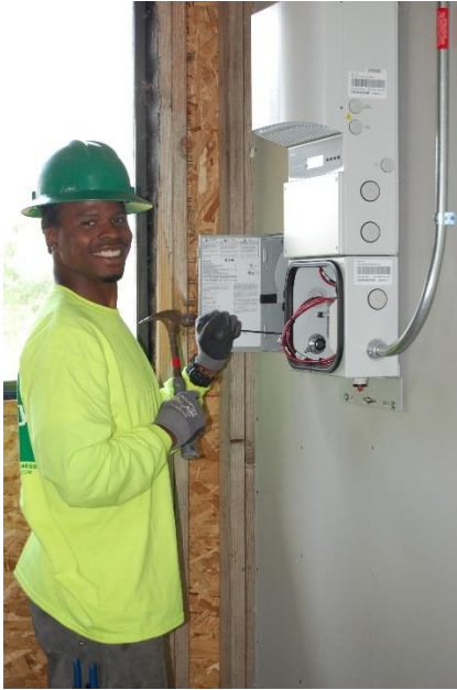
Installation of Aurora inverter, May 15, 2013
