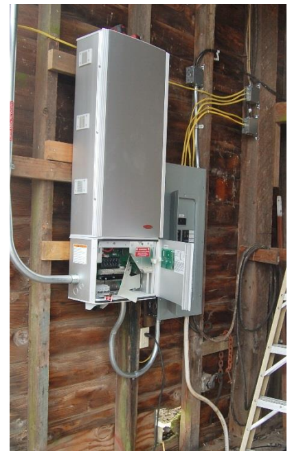
Check out the old meter and new inverter and meter base in the equipment barn.
