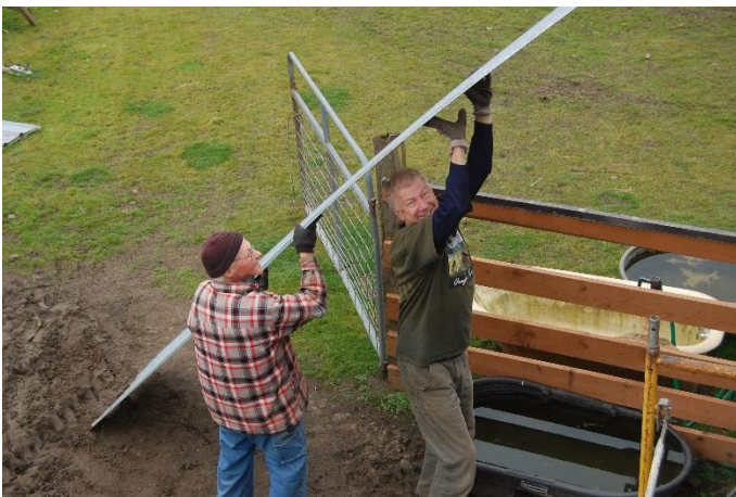
Ken and Phil hand up the metal roofing to Luke...
