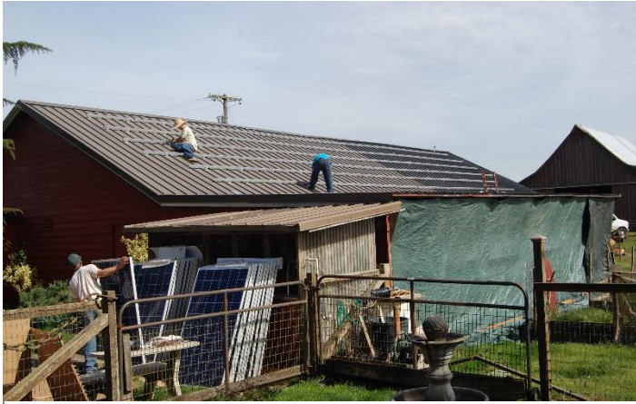
Solar Ki's crew install Unirac SolarMount racks onto the equipment barn.
