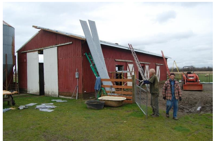
...and Luke screwed the metal roof; overlapping shorten pieces with the old metal roof.
