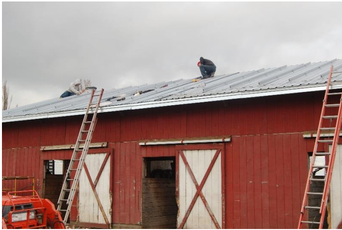
Laura's crew installed Unirac SolarMount racks on the roof.
