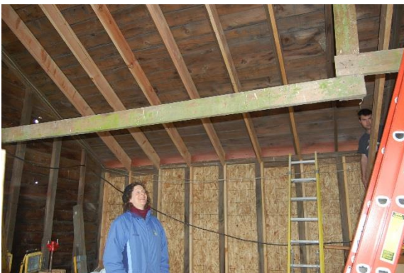
Interior of horse barn. 2X4's added lengthwise on the barn roof.
