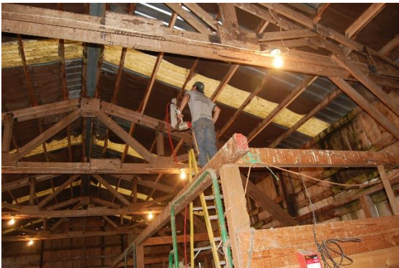
Interior of horse barn. 2X4's added lengthwise on the barn roof.
