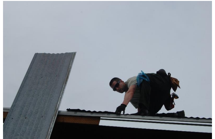
...and Luke screwed the metal roof; overlapping shorten pieces with the old metal roof.
