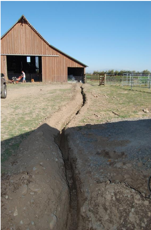
Underground line to the horse barn from the new meter base.
