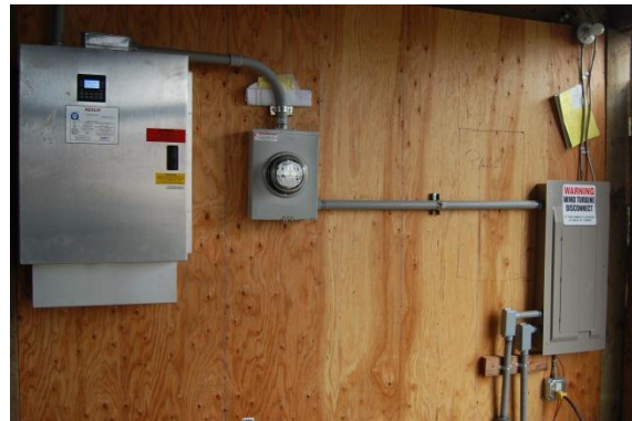
Inverter, meter base and hook up to turbine.
