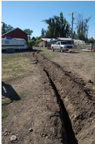
Underground line to the horse barn from the new meter base.
