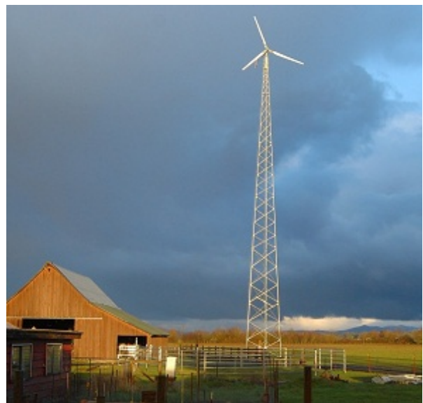
20-kilowatt wind turbine at Santiam Valley Ranch
